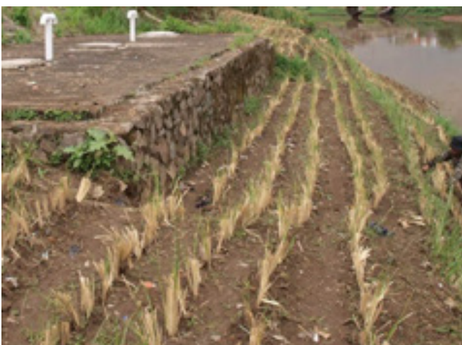
April 2009: Site is cleared and planted with 40,000 vetiver slips
